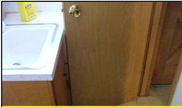
Basement bath door: replace sink with one less deep so door can swing freely?
