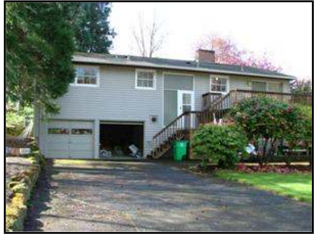
South face (fronts alley)
