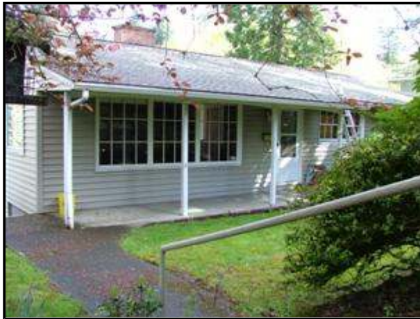
North face (front of home)
