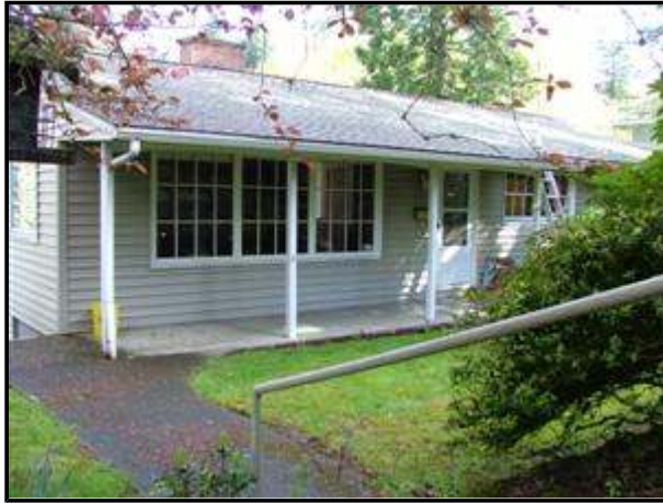
North face (front of home)
