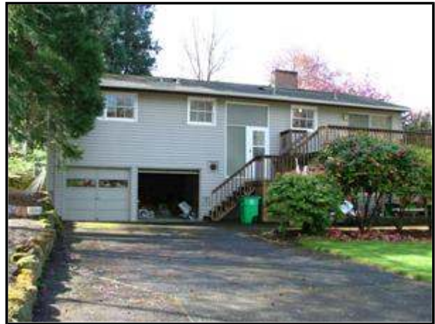
South face (fronts alley)
