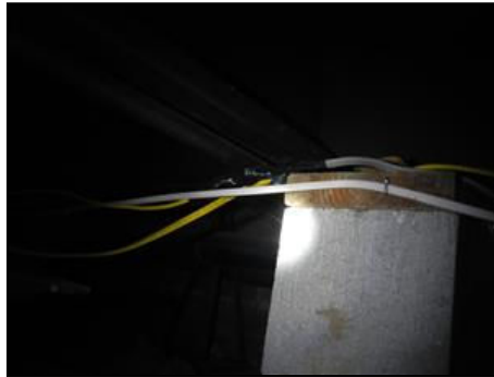
7.2 Picture 1 Improper wire splice in crawl space
