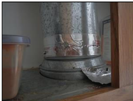
9.4 Picture 1 Connection of range hood with duct
