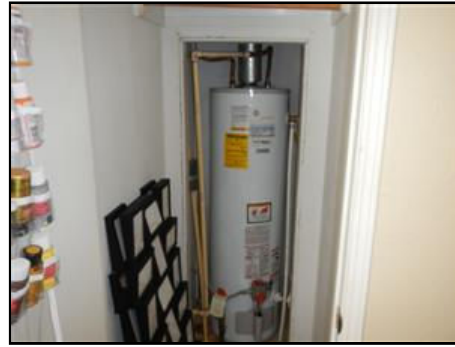
6.2 Picture 2 Water heater in alcove inside closet
