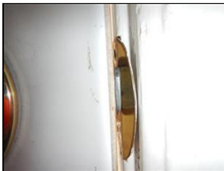
2.1 Picture 1 Deadbolt too high for strike plate in back door
