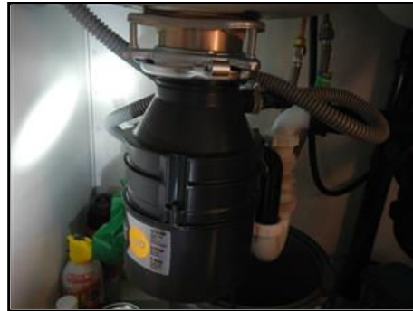
6.0 Picture 2 Garbage disposal with capped-off dishwasher drain hose attached
