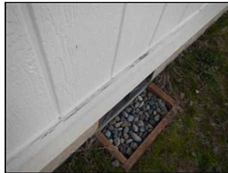
2.0 Picture 2 Paint peeling at top of trim board
