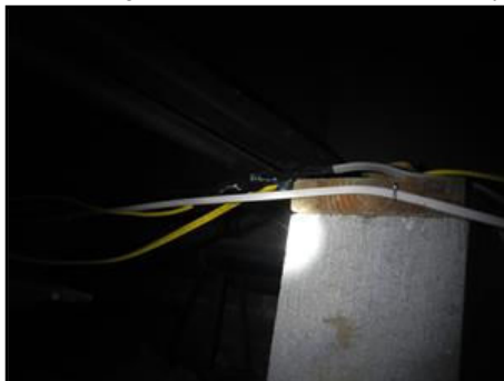
7.2 Picture 1 Improper wire splice in crawl space
