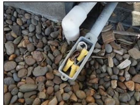
7.2 Picture 2 Conduit from crawl space at back of house (pull box cover removed)
