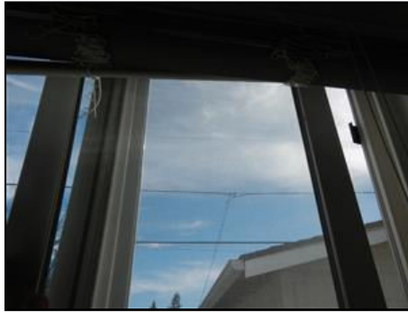
2.2 Picture 1 Laundry area window loose in track
