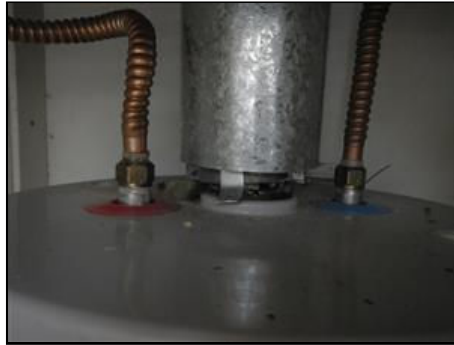
6.2 Picture 1 Hot water heater flue not attached
