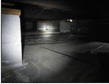
5.0 Picture 3 Efflorescence at bases of concrete block piers
