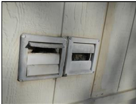
2.6 Picture 1 Dryer duct outlets
