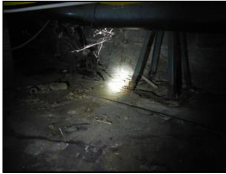
5.0 Picture 5 Ground anchor to left of recessed perimeter pier
