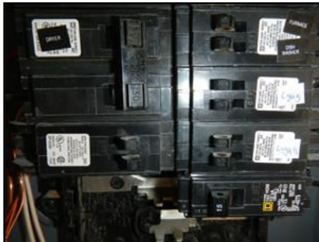
7.1 Picture 1 No identification for breaker in lower right
