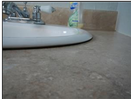
6.1 Picture 1 Sealant missing where bathroom sink meets counter
