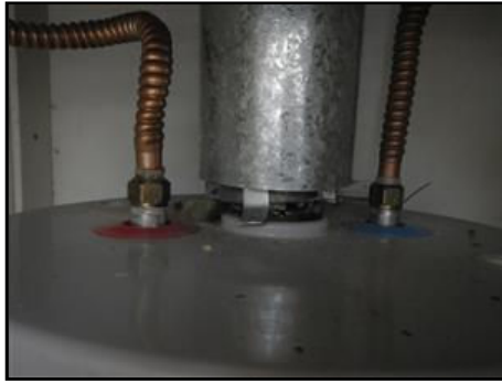
6.2 Picture 1 Hot water heater flue not attached
