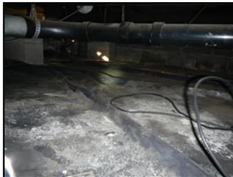
5.0 Picture 1 Signs of frequent water entry into crawl space
