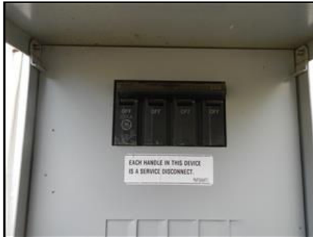
7.6 Picture 1 Main breaker at exterior meter panel
