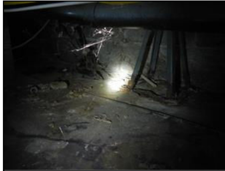
5.0 Picture 5 Ground anchor to left of recessed perimeter pier
