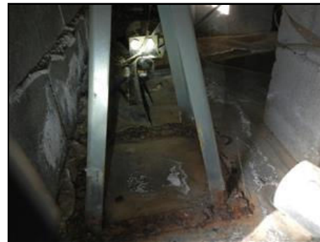
5.0 Picture 2 Rusted base of steel recessed perimeter pier
