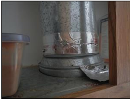
9.4 Picture 1 Connection of range hood with duct
