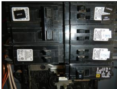
7.1 Picture 1 No identification for breaker in lower right
