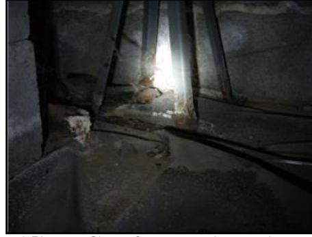
5.0 Picture 4 Signs of water entry into crawl space
