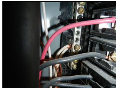
7.1 Picture 2 2 neutral wires in same lug
