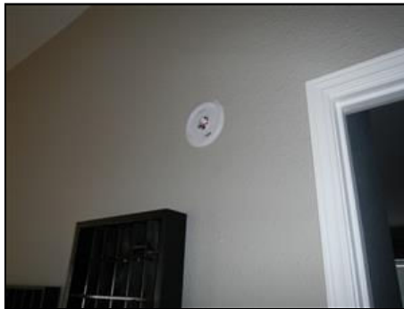
7.7 Picture 1 Bracket for smoke alarm on south side
