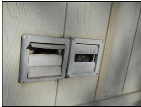
2.6 Picture 1 Dryer duct outlets
