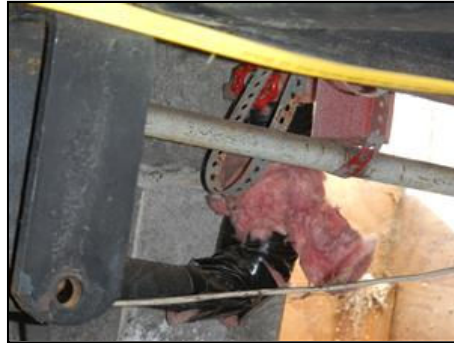
6.3 Picture 1 Red-handled main water shutoff inside crawl space
