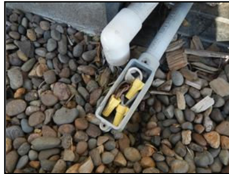
7.2 Picture 2 Conduit from crawl space at back of house (pull box cover removed)
